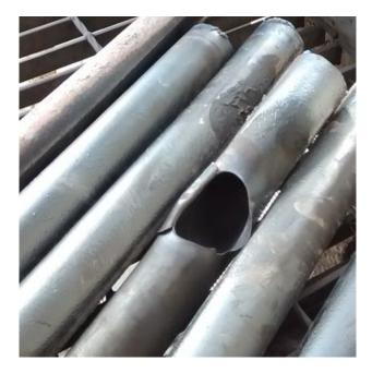
Welding workers immediately removed the defective tube by cutting and replacing it with a fresh tube. The new tube was welded in the same proportion so as to minimise the difference at the welded joint.
